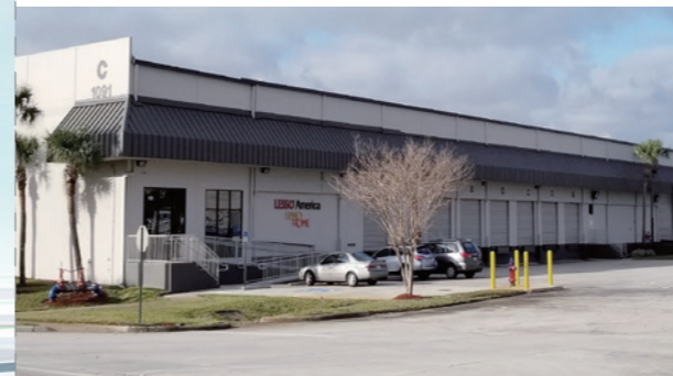
LESSO Florida Warehouse
